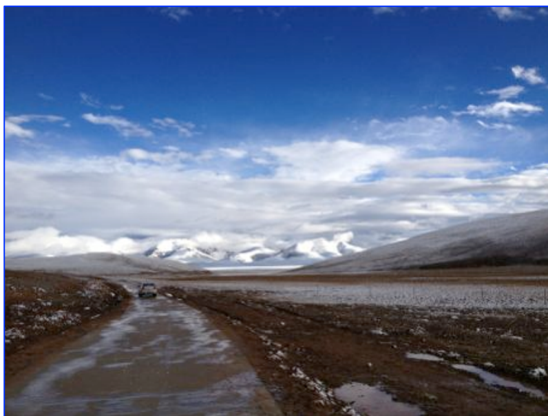
Newly-paved road to Rima
