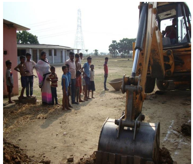
Let the construction begin!
