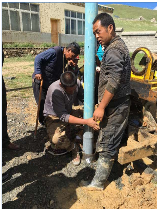
Figure 9 Inserting the PVC liner
