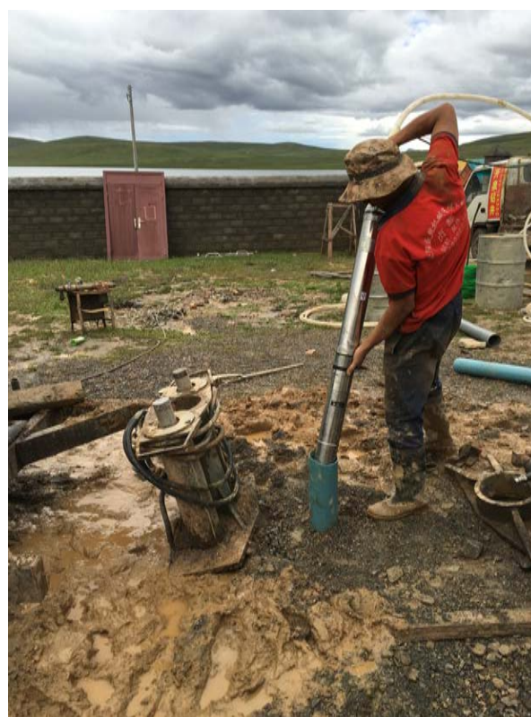
Figure 10 Inserting the pump
