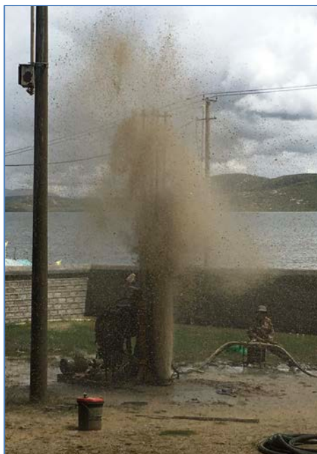
Figure 7 Striking water at 40 meters
